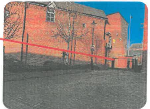
Side (rear) of Gardner Champion Solicitors where proposed bridge will be located.
