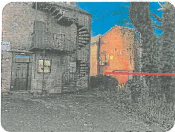
Side (front) of Gardner Champion Solicitors where proposed bridge will be located.
